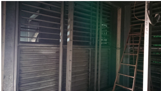
Photo: Shields Outside Air Dampers (Courtesy of ECO )
