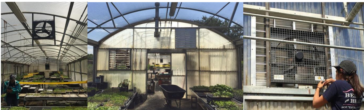
Picture 1: Middle-fan installed.
