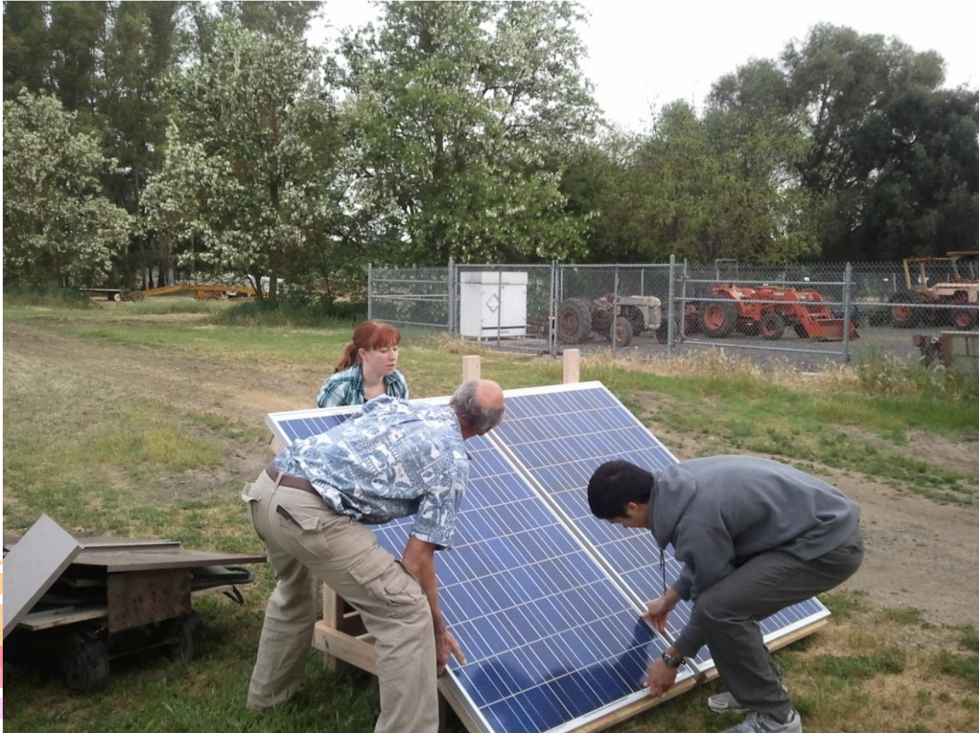
Install Solar Panel
