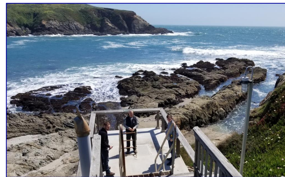
Figure 3: Pumphouse location pulling up to 1,000,000 gal/day of seawater
